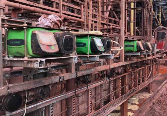
The heart of the Verderflex Vantage 5000 is its gentle, zero backflow peristaltic pumping action. This simple principle results in precise doses and accurate flows.
